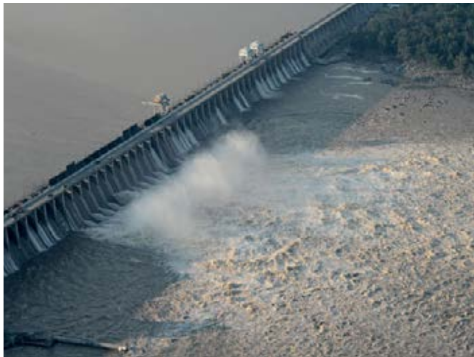
Sediment and phosphorus being scoured through the Conowingo Dam following Tropical Storm Lee in September 2011.
