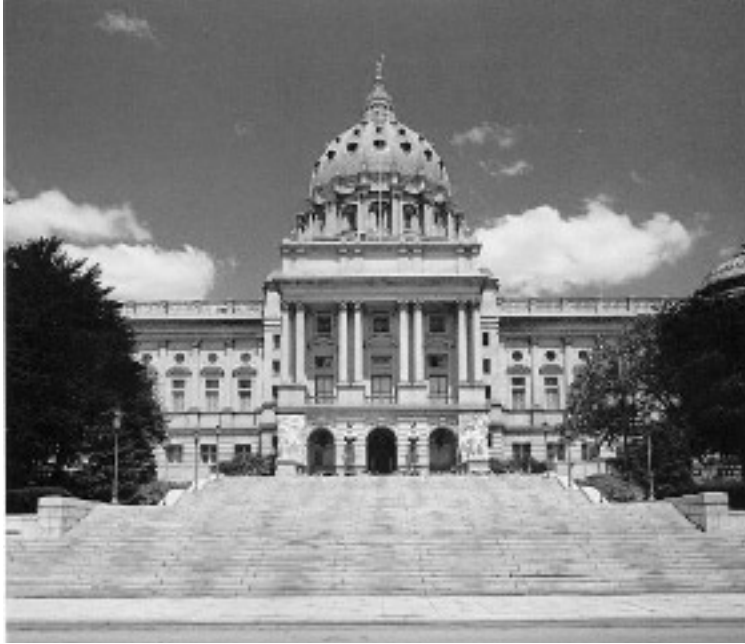
The State Capitol Building: Harrisburg, Pennsylvania
