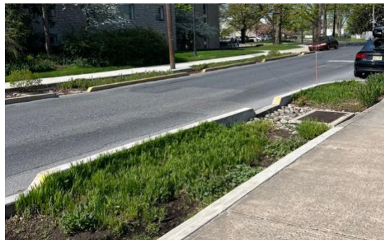
Bioretention, West Louther St.
