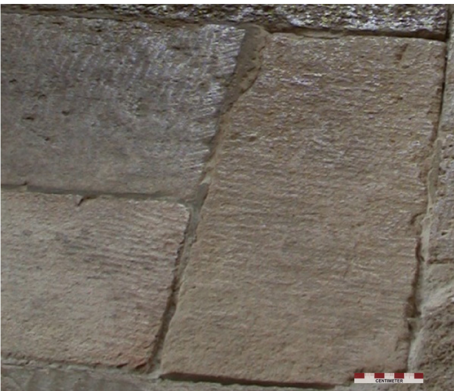
Figure 2. Parallel tool marks on the surface of Purbeck Stone pavers from the floor of the nave of Christ Church.
