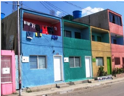
Houses built by community volunteers using a government grant
