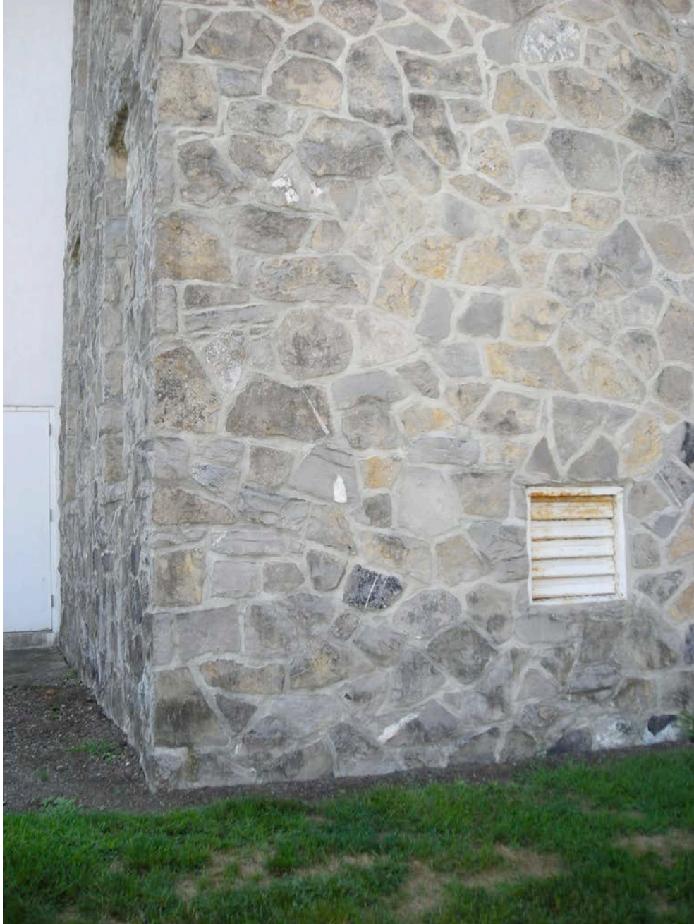
Stone in Kisner-Woodward is laid as irregular rubblework.
