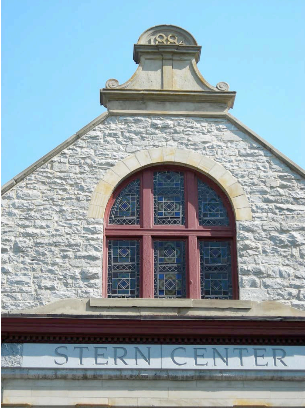
Front of Stern Center. Trim above and below window and below sign are made of Ohio sandstone. Stern Center sign is made of granite, which replaced an older sign made of granite that said "Scientific Building."
