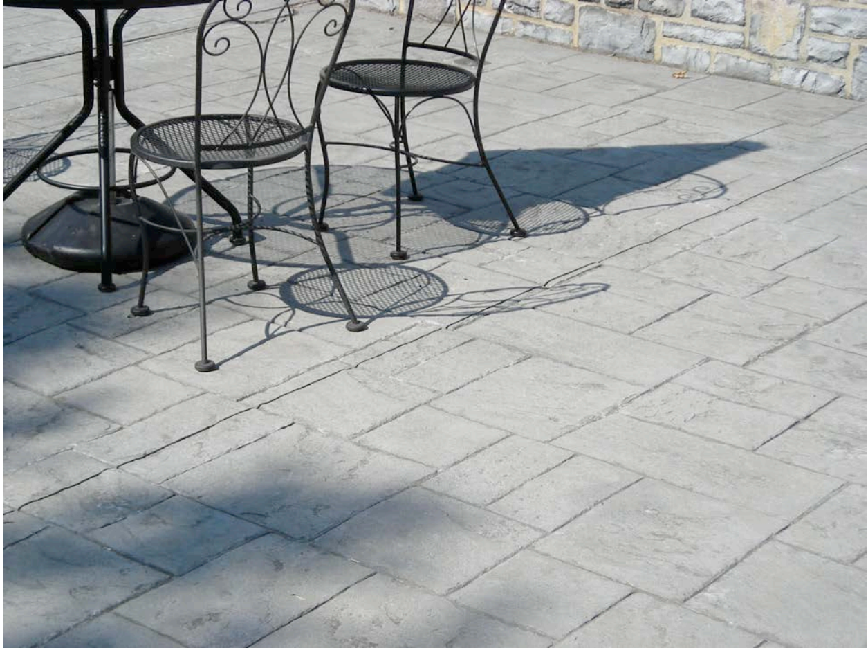
Stern Center patio looks like it has bluestone pavers, but don't be fooled. The "pavers" are poured concrete, which is then stamped with a pattern to make it look like real stone.
