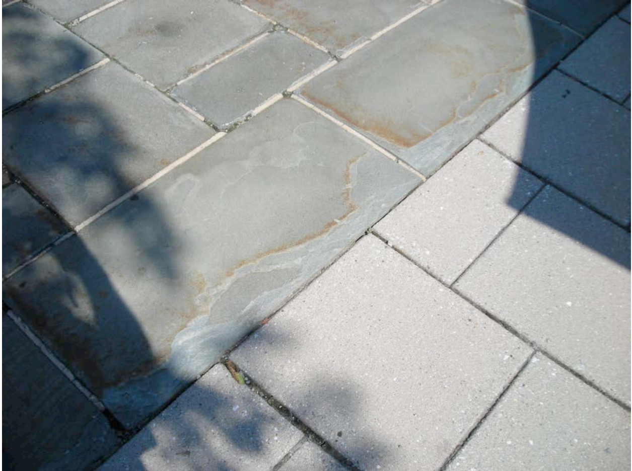
Patio in front of Weiss Center is made of Pennsylvania bluestone (upper left) and artificially made cement pavers (lower right). Note how the bluestone spalls or flakes (near junction between materials).
