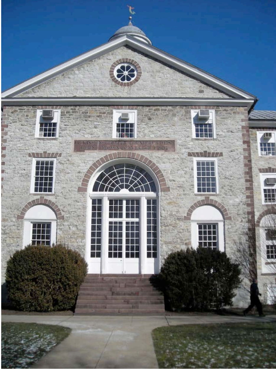
Old West, showing details of red sandstone trim in arches and keystone blocks over windows, steps, and quoins (trim at corners of building).
