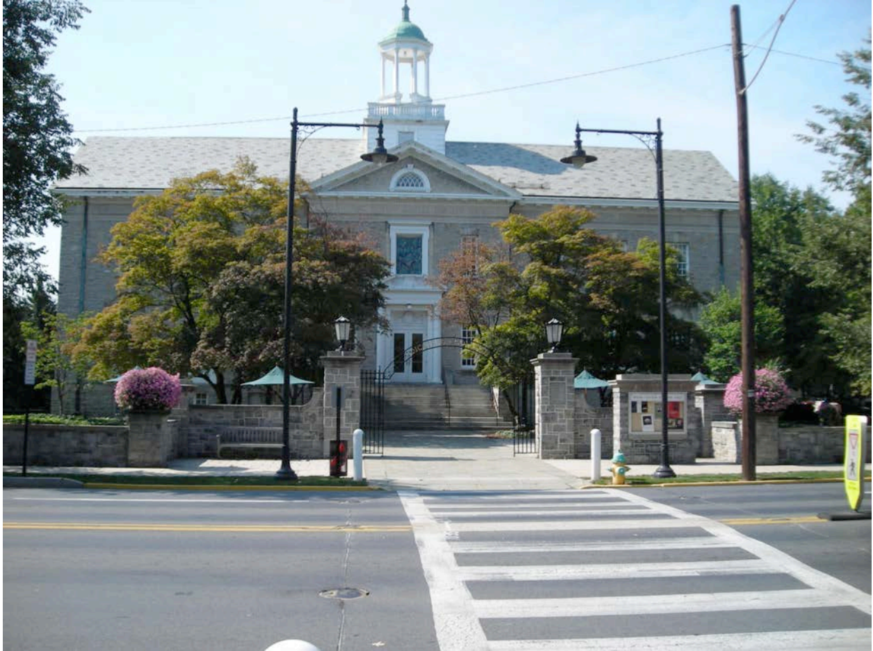
Weiss Center for the Arts, originally Alumni Gymnasium opened in 1929, renovated as Weiss Center in 1983, is made of local limestone.
