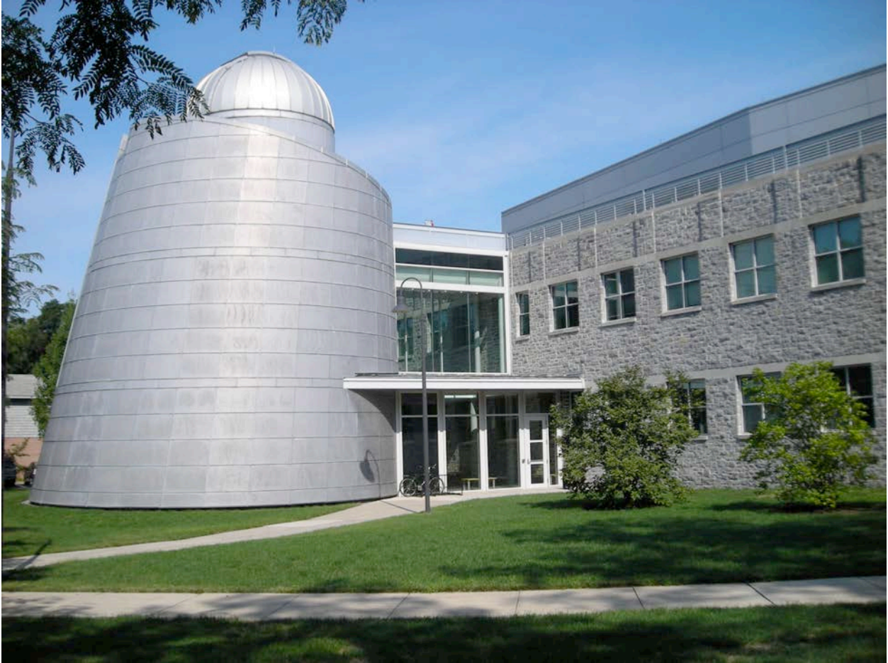
The stone in Tome Hall (2000) is Ordovician limestone that was quarried at the Dickinson College Quarry west of Carlisle near Plainfield.
