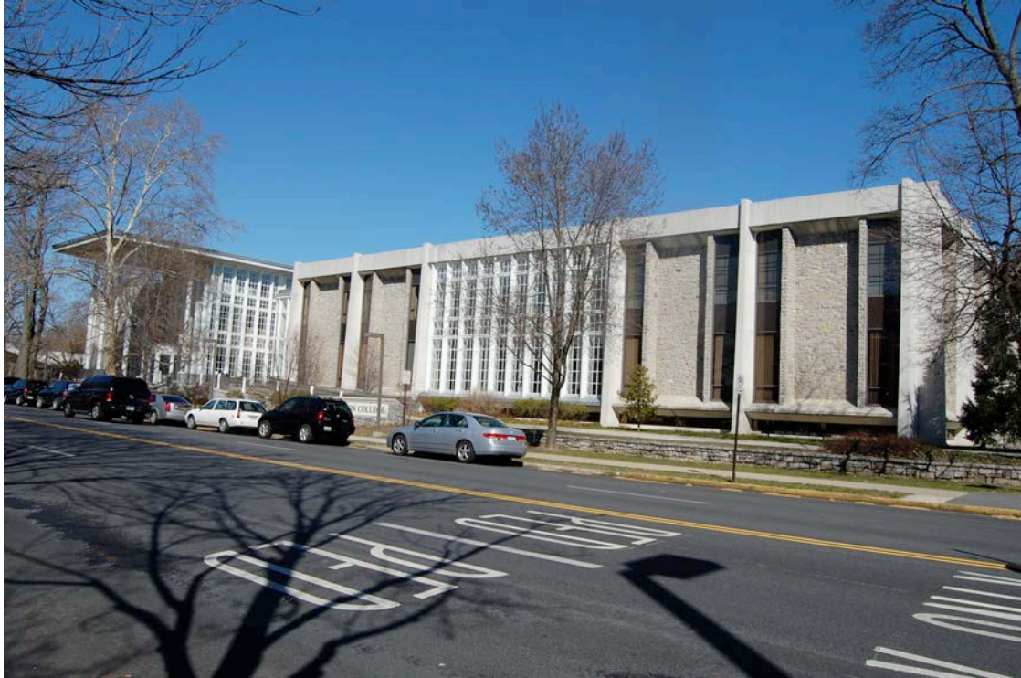
Spahr Library (1968) panels between windows are made of local limestone. Original entrance was where the mullioned windows are today.
