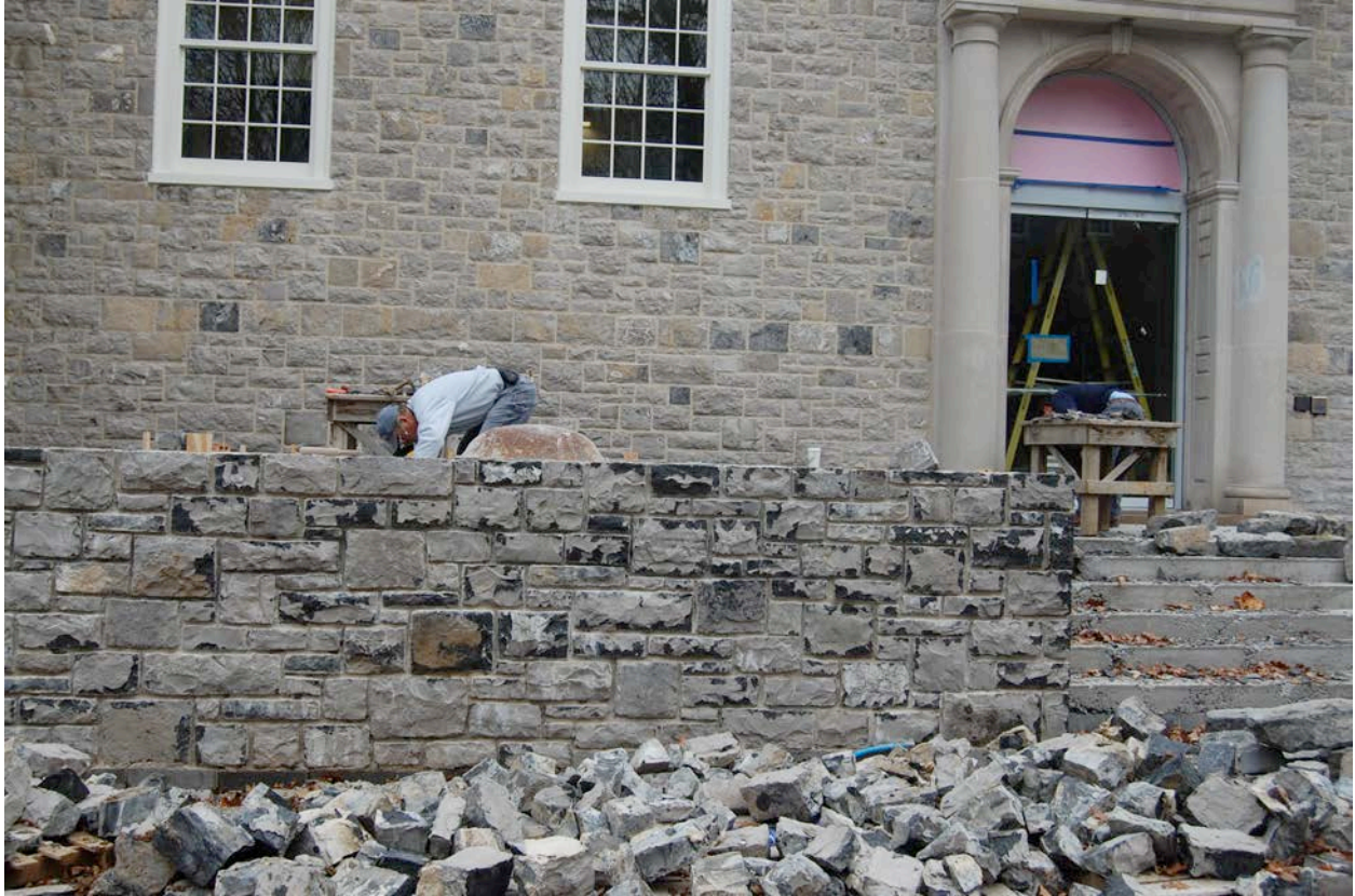
11/5/2009—The new porch on Althouse takes shape. The limestone in the foreground will be sandblasted to make it look old and light gray.
