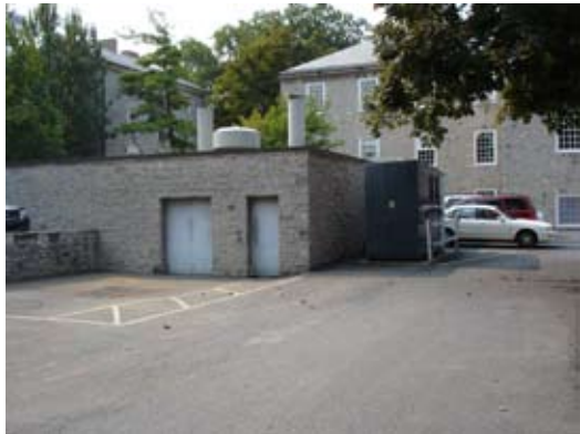
1 The central heating building
