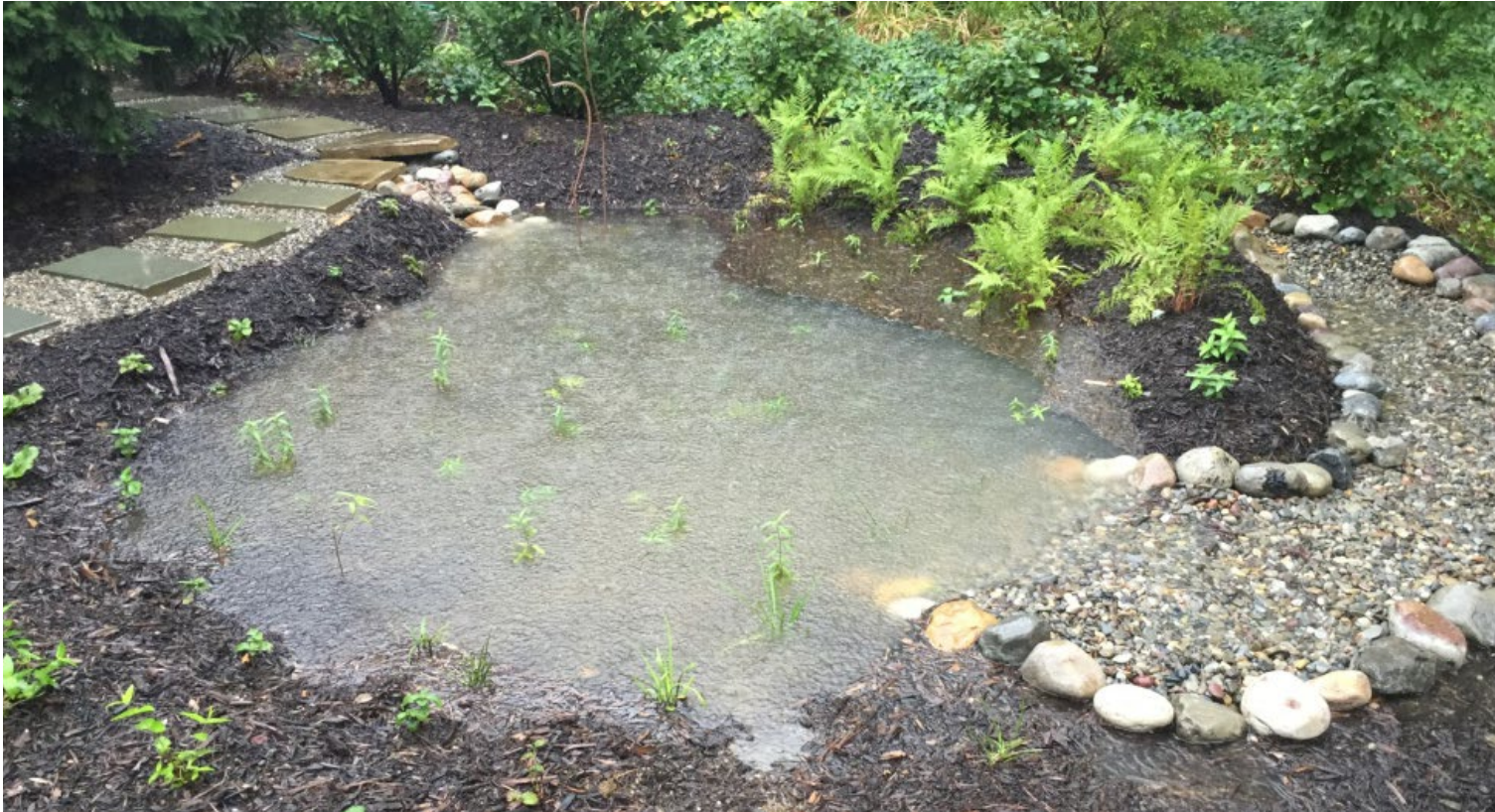
A residential rain garden filled after a storm in Lancaster, PA (Photo courtesy Lancaster County Conservancy).
