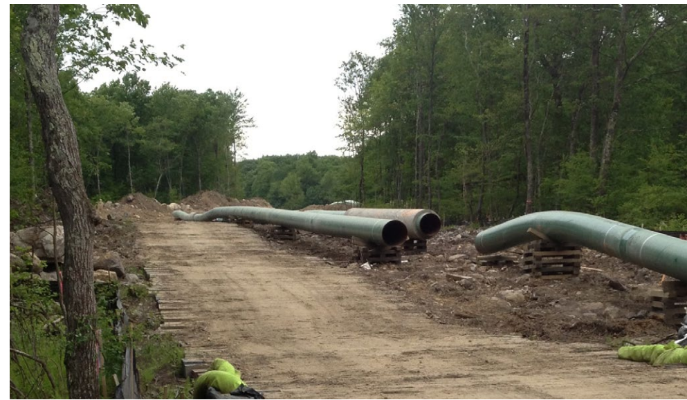
Pipeline installation in progress (Photo courtesy Delaware Riverskeeper Network).
