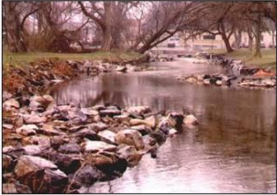
Stone deflectors to increase rate of flow and decrease sedimentation
