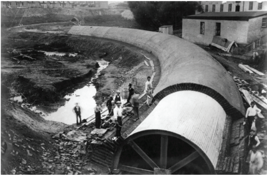
Mill Creek Sewer, West Philadelphia, ca. 1883. This sewer, constructed over five miles, obliterated the largest waterway in West Philadelphia for which it is named. Much of Philly's sewer system is over one hundred years old and suffers its age. Retrieved from http://www.phillyh2o.org/
